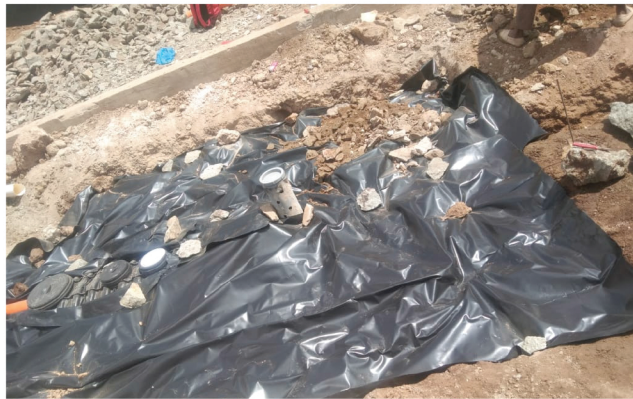
Step 5: Cover the soaking pit with dump proof membrane (black polythene)
